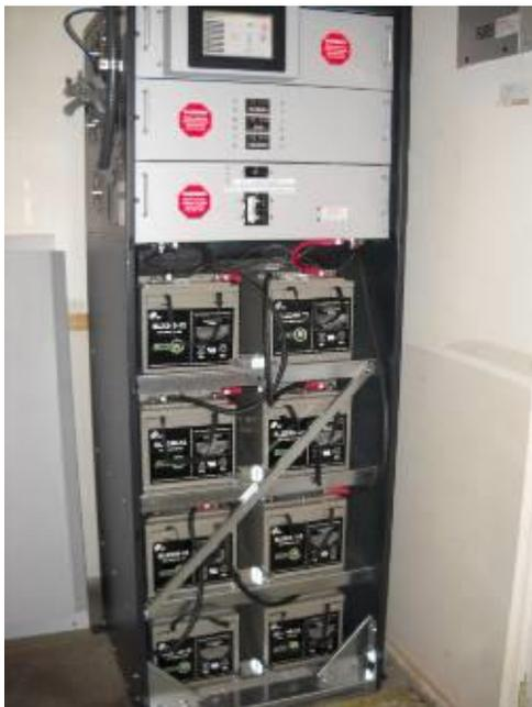
**Figure 2. 9-kW SP Unit with Cover Removed**
