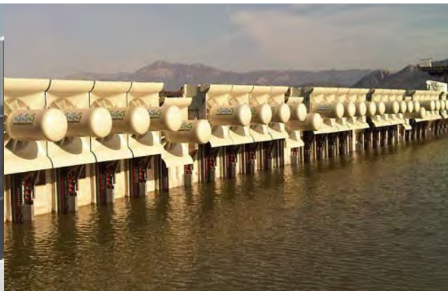
Figure 1-10. Modular application of standard turbine runners to an existing dam
