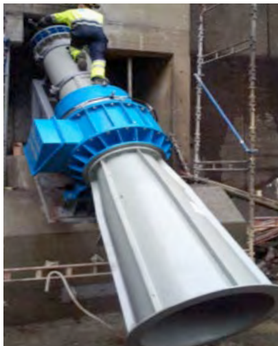
Figure 1-11. Inclined (left) and horizontal (right) integrated turbine-generator technology installed without a powerhouse
