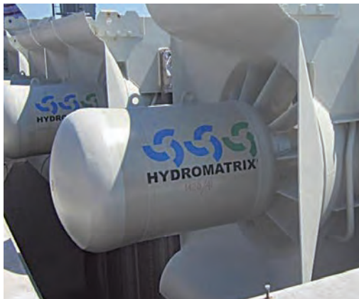
Figure 1-10. Modular application of standard turbine runners to an existing dam
