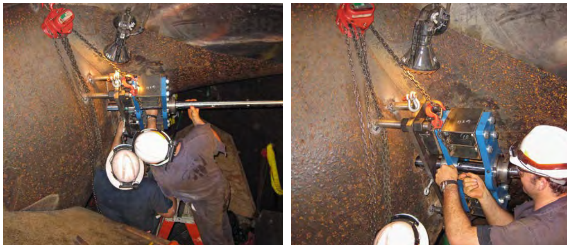
Figure 2-52. Final adjustments of line boring equipment for installation of new turbine blade dowels
