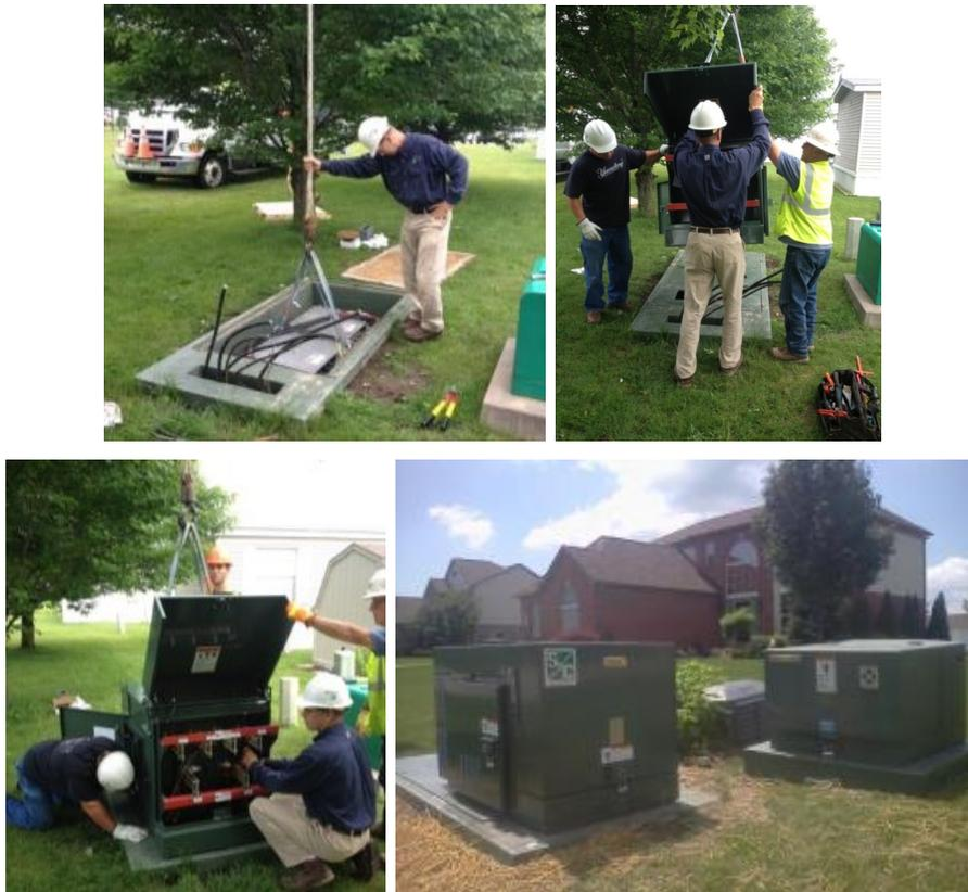
Figure 10: DTE CES system installation. In the bottom right photo, the CES is located to the left and the transformer is located on the right [9].
