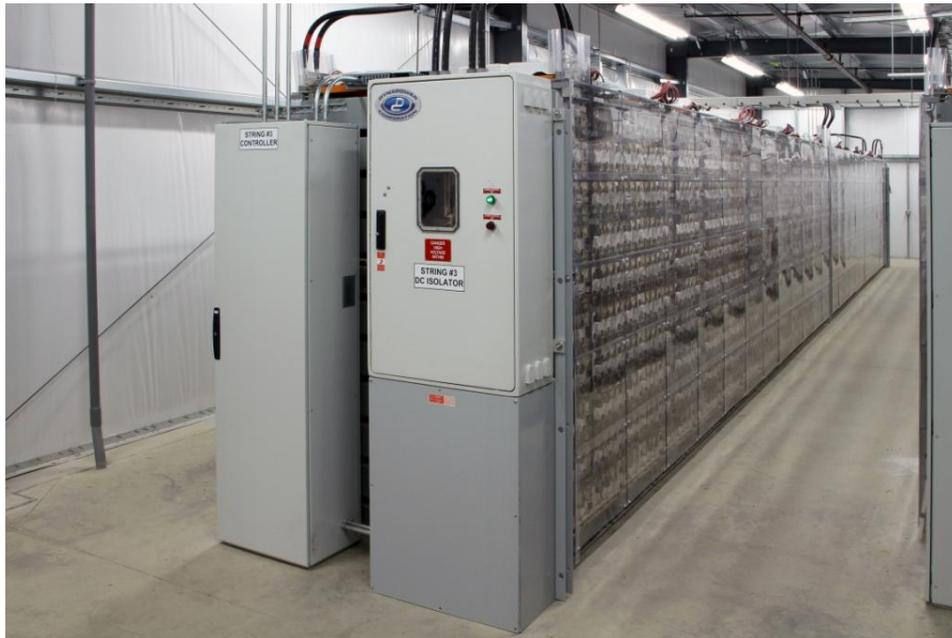
Figure 3: East Penn UltraBattery installation [3].
