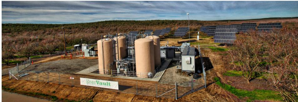
Figure 8: EnerVault Fe-Cr Redox flow battery, Turlock, [7].
