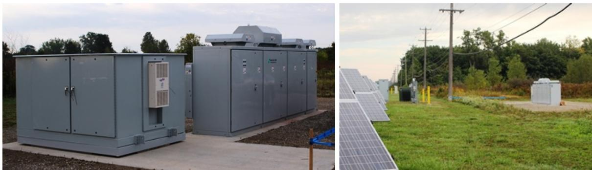
Figure 11: DTE 500 kW system collocated with a 500 kW PV [9].
