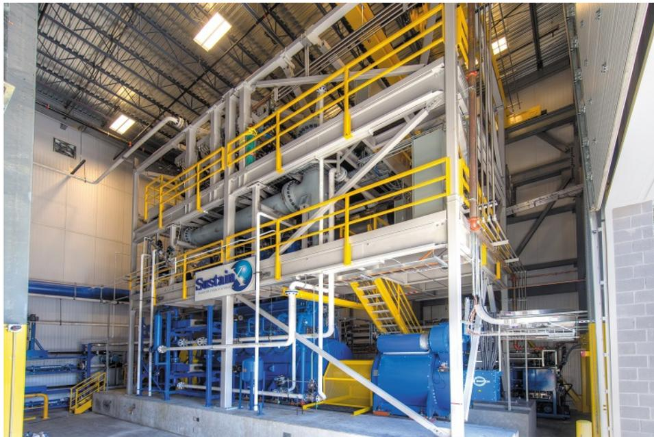
Figure 12: SustainX 1.65 MW isothermal CAES.
