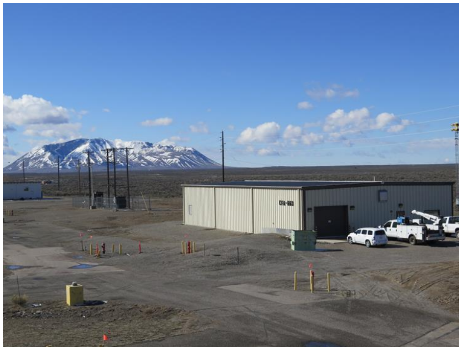
Figure 2. CSL exterior view.
