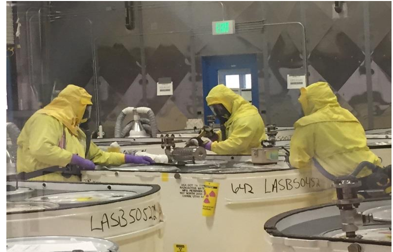
Workers install pressure relief devices
