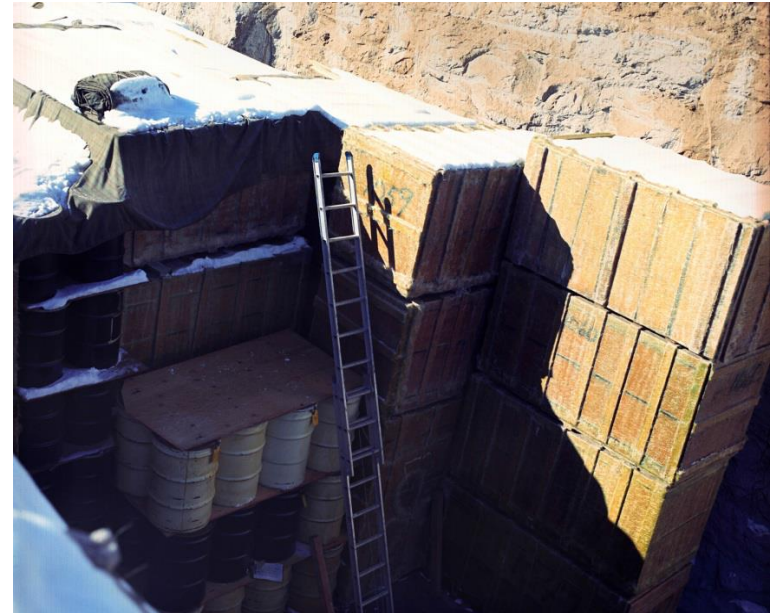
Retrievable TRU waste (drums & boxes) in Pit 9
