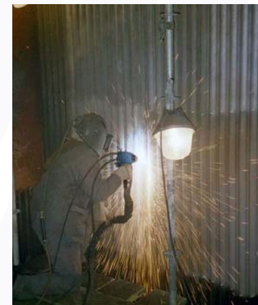
On site Coating of a coal boiler waterwall www.thefabricator.com
