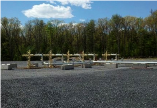
Figure 2. Typical Marcellus well pad with multiple adjacent trees (GoMarcellusshale.com)
