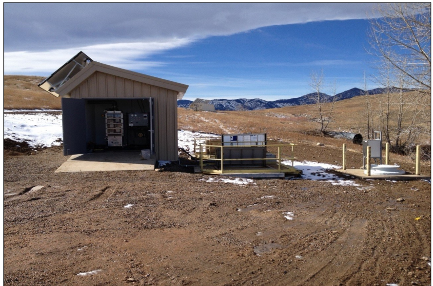
Rocky Flats Air Stripper with Solar Power
