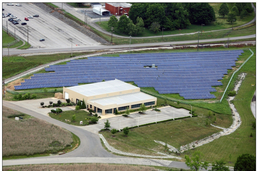
Powerhouse Six 1 Megawatt Solar Farm at the ETPP in Oak Ridge, Tennessee
