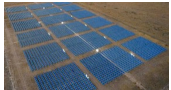
Tucson Electric Power, NREL 13327
