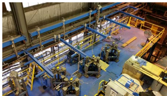
Mechanisms Engineering (Sodium) Test Loop at ANL
