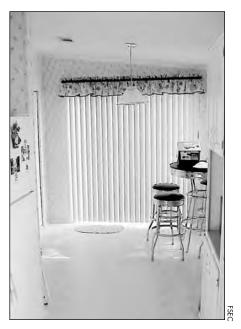
This kitchen has a vinyl floor covering and an overhead supply register. Mold can occur under the vinyl that is washed by cold air from the register.
