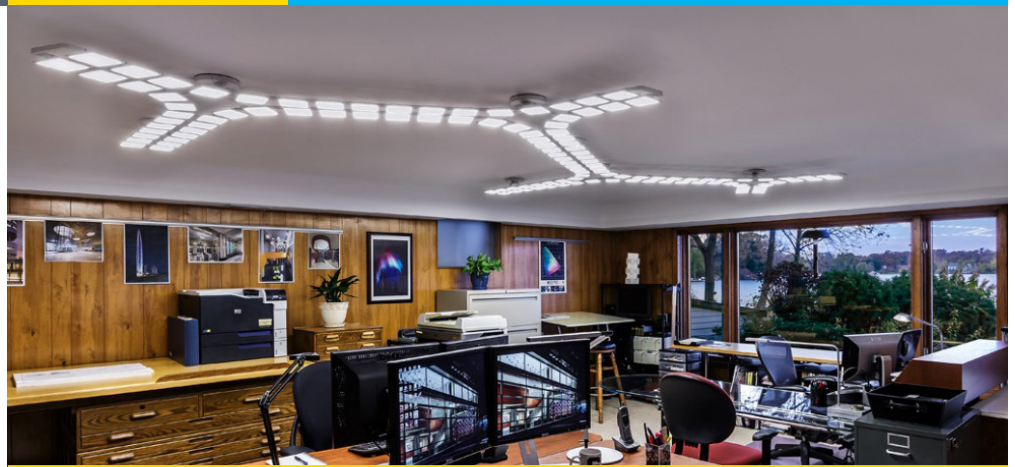
The office of Aurora Lighting Design, Inc., with its lighting system using OLED panels. Photo courtesy of Acuity Brands.
