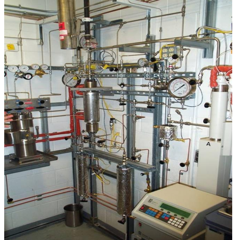
PNNL bench-scale, continuous-flow, fixed-bed, catalytic hydrotreater
