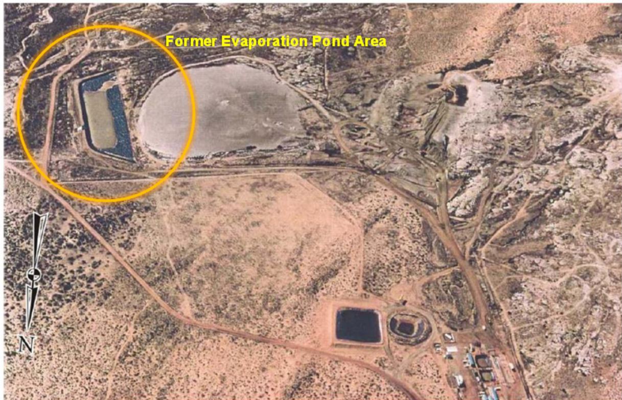
Figure 3. Evaporation Pond at the Monument Valley Site During Milling Operation (March 1993) Photo is from the 2010 assessment (DOE 2010). Note orientation of north arrow.
