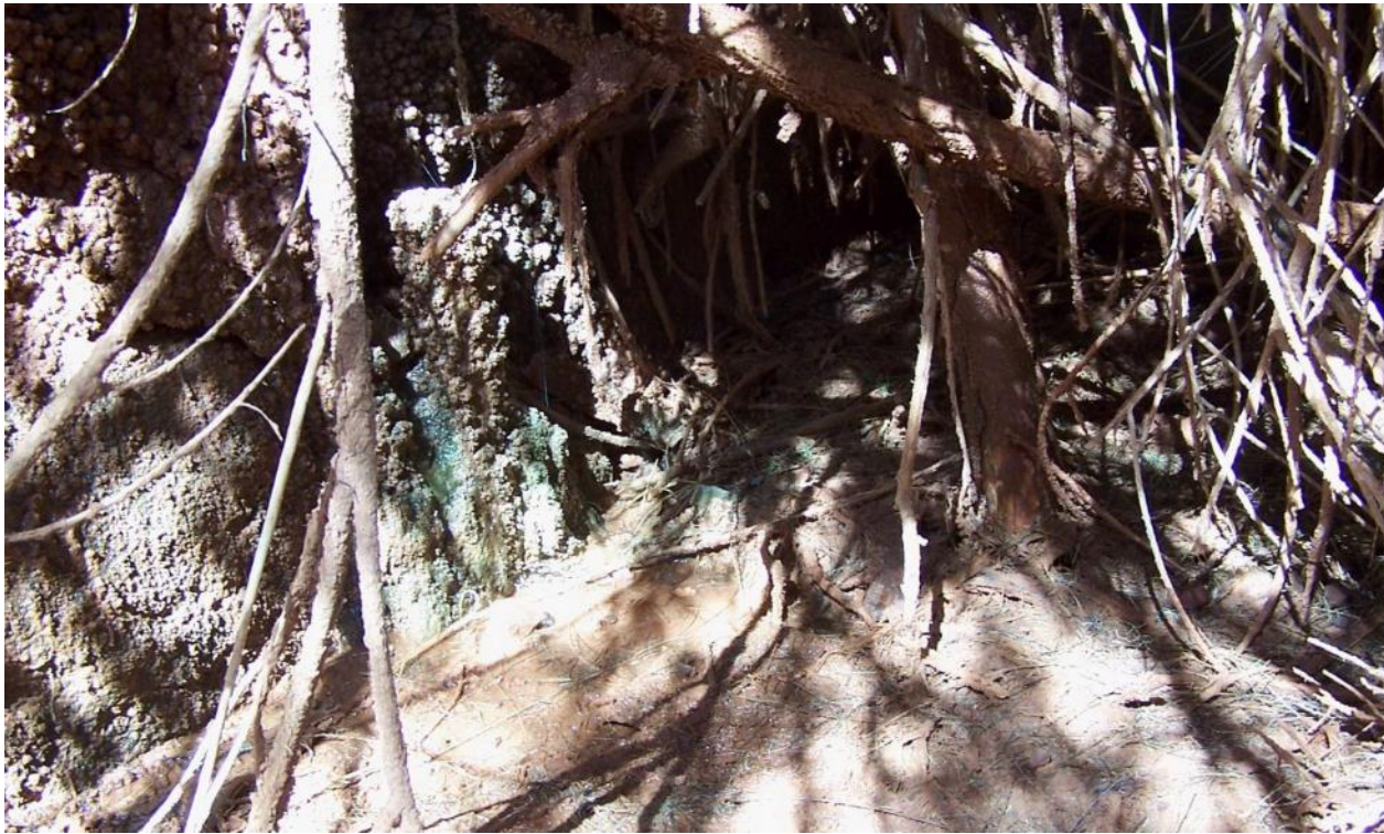
Figure 24. Mexican Hat, Utah, 2006 Photos of Formation of Evaporite Deposits Along Seep 0248
