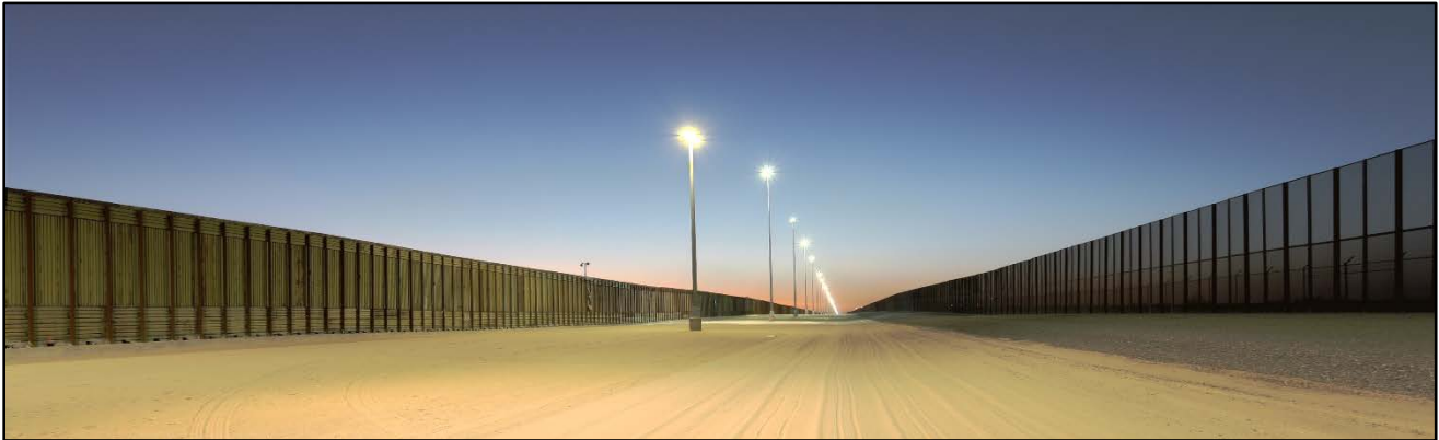
Figure 1. Trial Demonstration Site on the U.S.-Mexico Border. Photo taken looking west from the east end of the 7.2 mile area between poles 204 (not pictured) and 203 (pictured, front). The QMH luminaires are mounted on the poles at a height of 64 ft and the LED luminaires are mounted at 40 ft—a difference that is visible in this image. The primary fence is on the left and the secondary fence is on the right.
