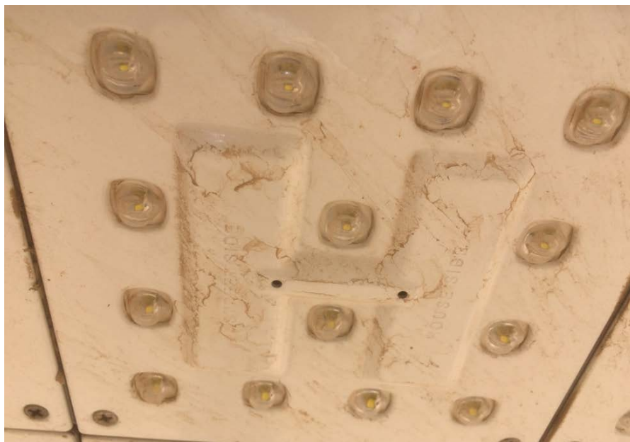
Figure 18. Dirt Accumulation on Luminaire A. This photograph was taken by the electrician prior to removing the luminaire.
