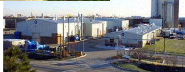
Energy & Environmental Technology Center
