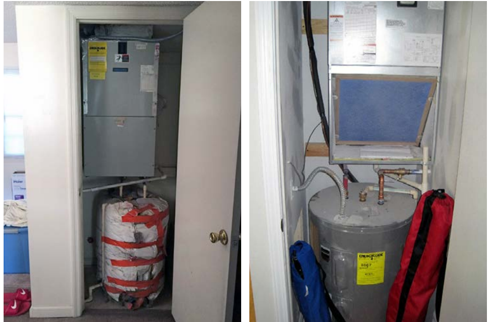
HVAC systems in the pre-rehabilitation (left) and post-rehabilitation (right) conditions. Rea Ventures upgraded the heating and cooling efficiencies and access to the filter for easier inspection and maintenance.
