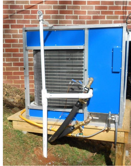
Alpha 2 Field Test (combi) (GTI Monitoring)
