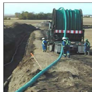
Figure 1. Installation of a spool of FRP.
