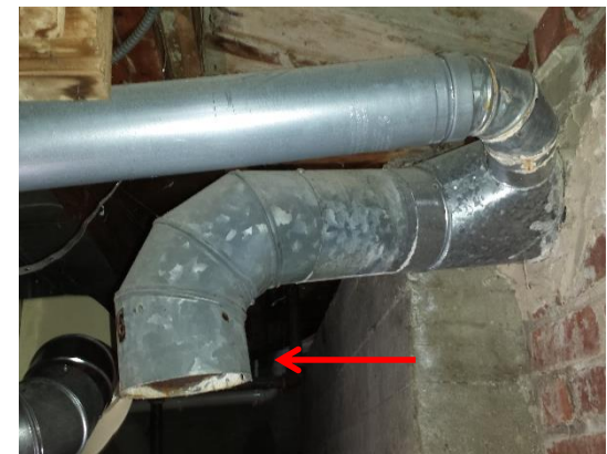
Water heater and unused furnace vent
