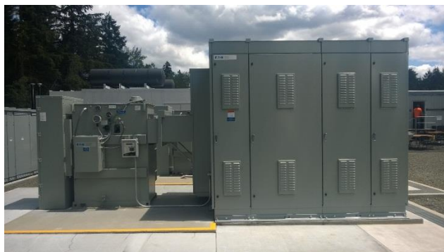
Representative outdoor breaker and control equipment (Courtesy Eaton)
