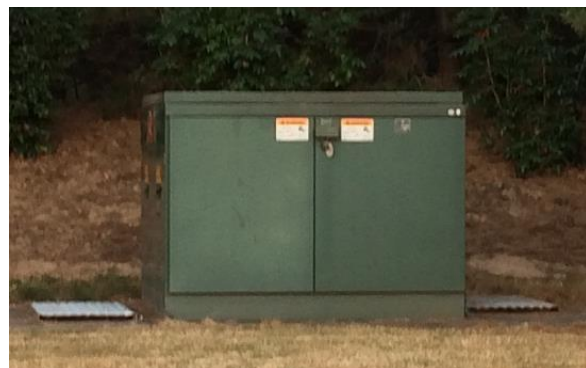
Typical of sectionalizing switch
