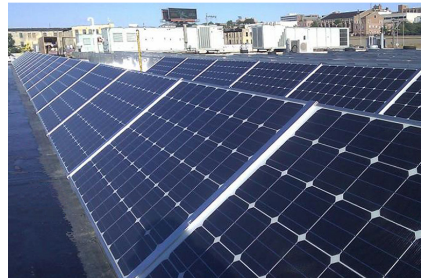
The Forest County Potawatomi Tribe's 30-kW solar PV system on the roof of its administration building in Milwaukee, WI. Photo from the Forest County Potawatomi Tribe, NREL 20107.
