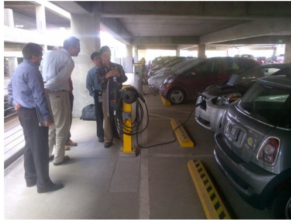
Figure VI-152: NREL Demonstrates Interface between Vehicle and Building Energy Management Systems at NREL Parking Garage
