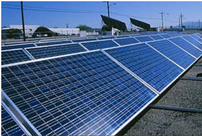
Tucson Electric Power's 300 KW PV Facility Adjacent to Its TEP Substation
