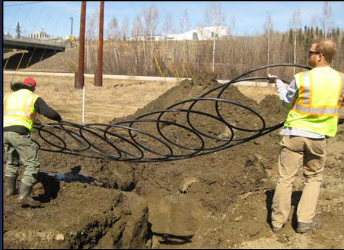
Installation of Slinky Loop
