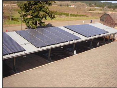
PV panels installed on Grand Ronde Tribal Housing Authority carport. 42 kW: Combination of tribal funds and state incentives Photo from GRTHA, NREL 31797
