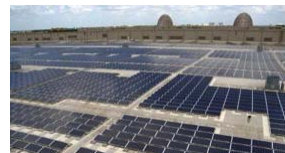
Orange County Convention Center, NREL 18077
