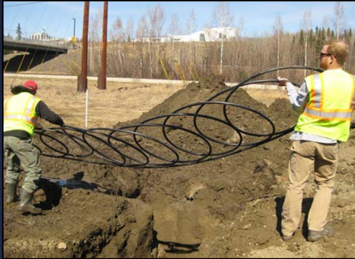
Installation of Slinky Loop
