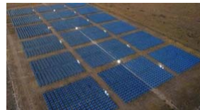
Tucson Electric Power, NREL 13327
