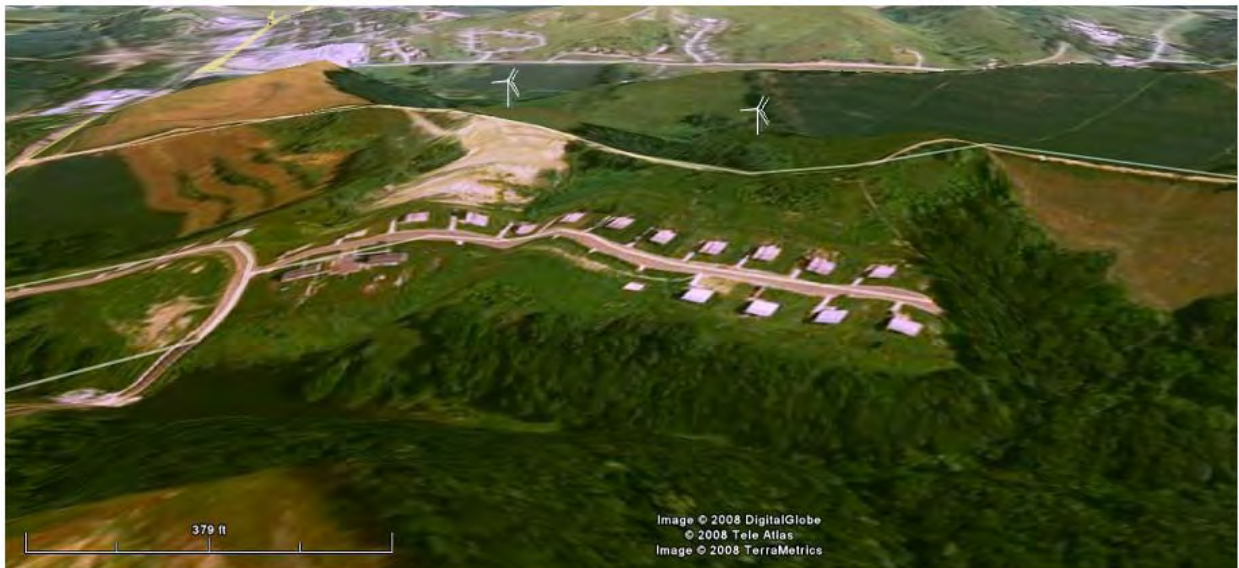
Figure 5.3-2, Kelly Subdivision, Northern View, Post-Construction
