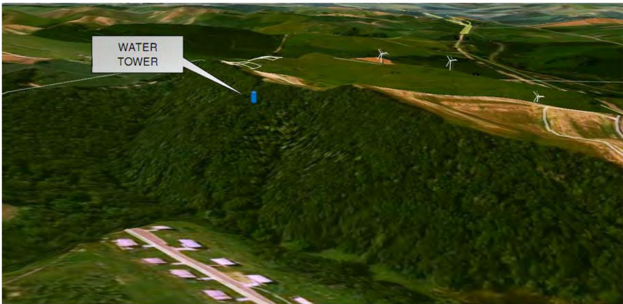
Figure 5.3-4, Kelly Subdivision, Southern View, Post-Construction
