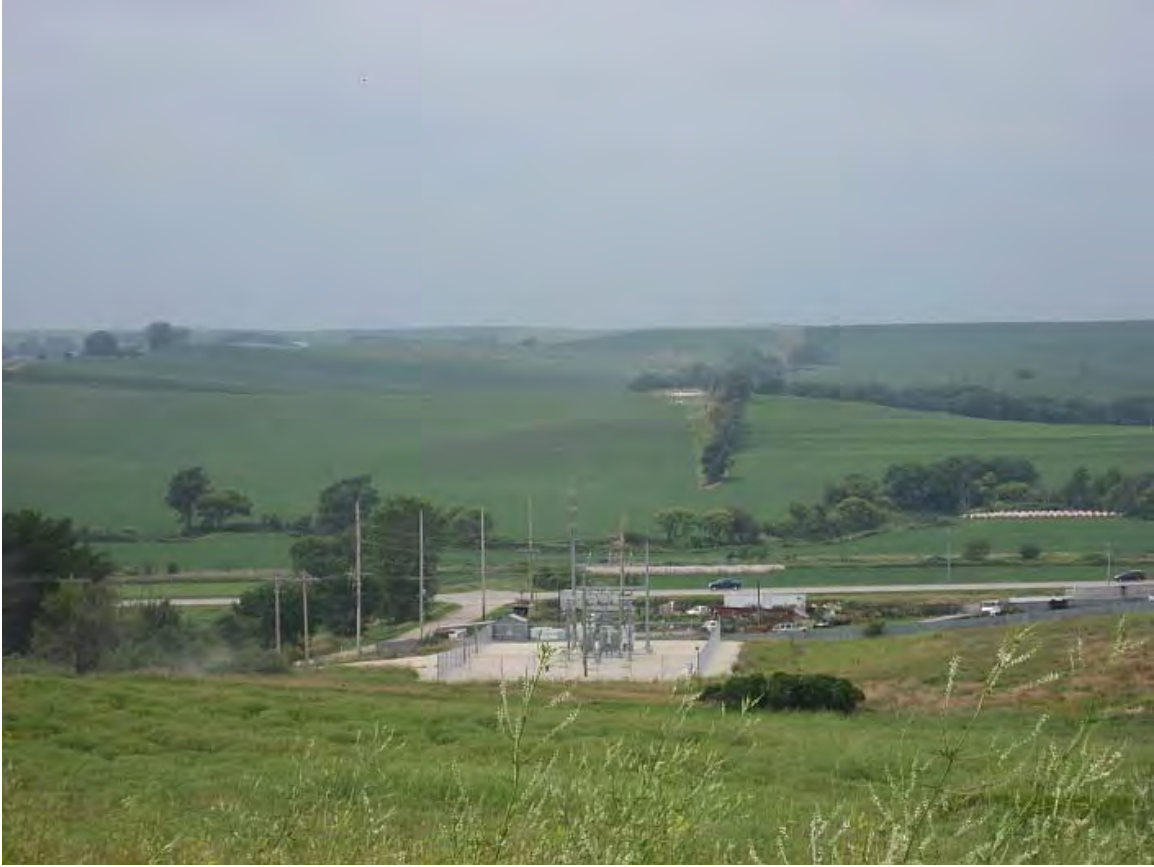
Figure 4.3-4, Looking West Toward Substation
