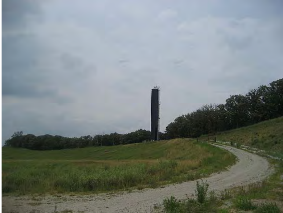
Figure 4.3-6, Looking North Toward Water Storage
