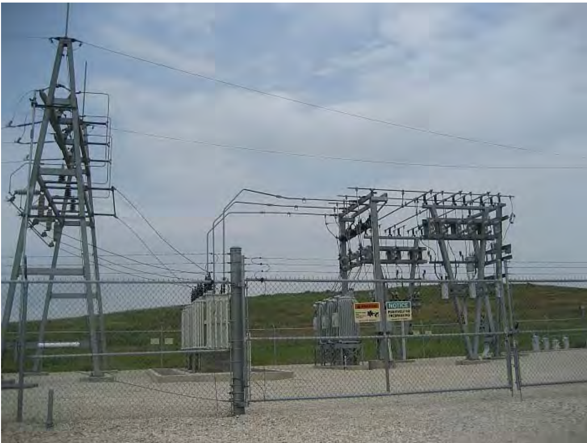
Figure 4.3-3, Looking North to Substation
