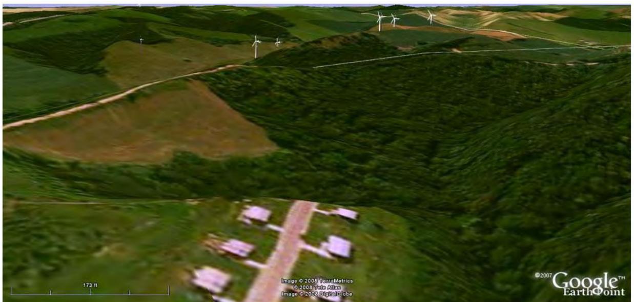
Figure 5.3-5, Kelly Subdivision, South East View, Post-Construction
