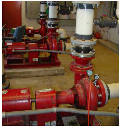
3 x 15 HP Lake Pump in New Hatchery
