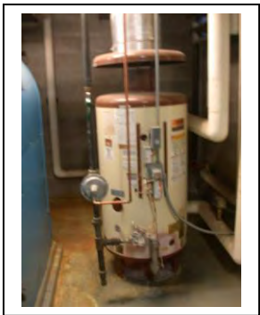
Propane Hot water in School Boiler Room
