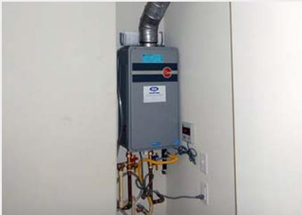
Instantaneous water heaters, even tank-type heaters, can be distributed among water-use zones to minimize water and energy waste.
