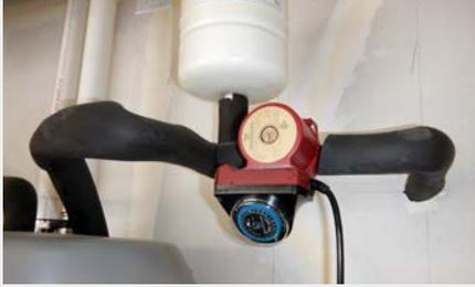
A simple approach is to add a circulation pump that senses a request for hot water. The main hot water must form a loop.
