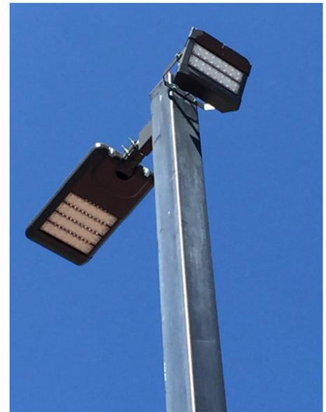
These low-wattage LED parking lot fixtures use only 133 W per lamp while the HID lamps they replace consume 1,080 W of input power per lamp.
