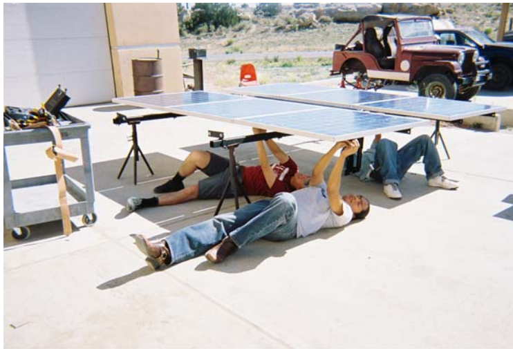
Figure 2: Sandia interns mounting the PV modules onto the sun tracker.
