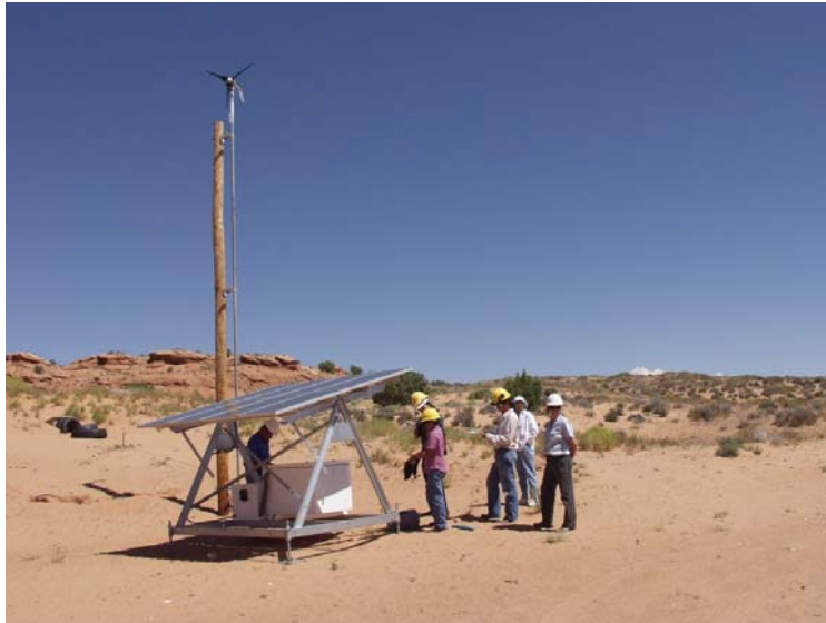
Figure 4: NTUA's PV and small wind hybrid unit.
