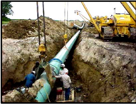
X52 or X65 Line Pipe (i.e. base metal)
