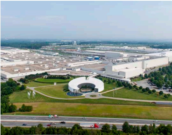
The BMW manufacturing plant in Greer, South Carolina. Landfill gas accounts for about 30 percent of the plant's electrical needs and about 50 percent of the plant's total energy requirements. Photo courtesy of BMW.
