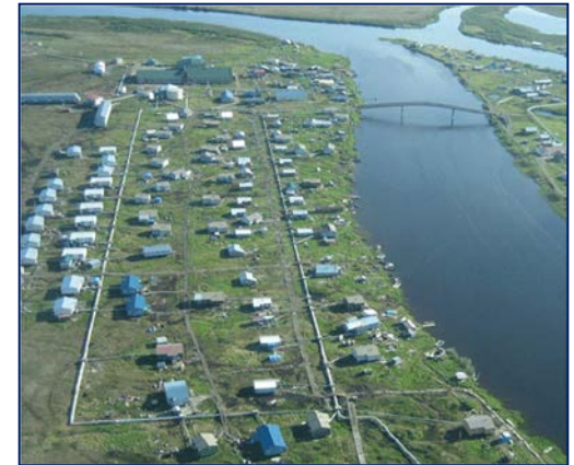
Alaska Native Tribal Health Consortium (Selawik, AK) will upgrade sanitation facilities
