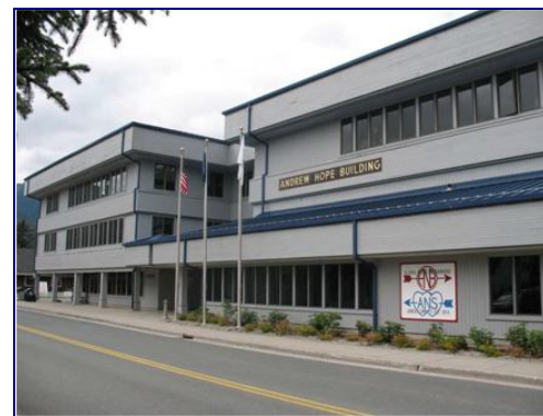
Central Council Tlingit & Haida Indian Tribes of Alaska (CCTHITA) retrofitting four buildings for projected annual savings of $52,271 (AK)
