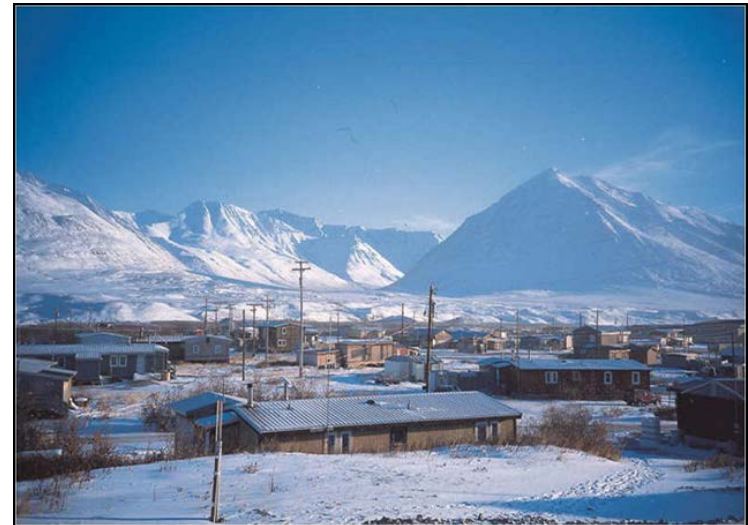
Yukon River Inter-Tribal Watershed Council (YRITWC) installed energy efficiency measures for the Nunamiut people of Anaktuvuk Pass to reduce energy use by 34%
