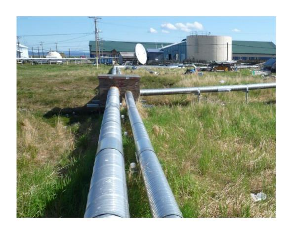
Photo 7: Junction box – reinsulation of these boxes improved efficiency
