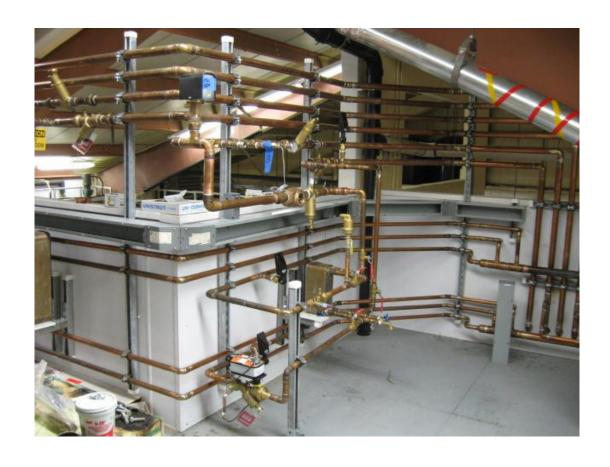
Photo 4: Hydronic heat add piping in the water treatment plant before insulation was installed
