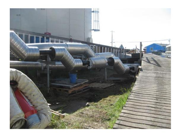
Photo 3: Vacuum sewer main (realignment and heat trace installation underway)
