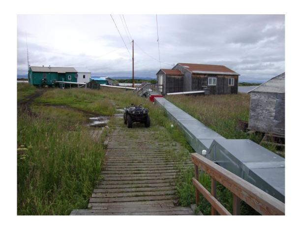
Photo 8: Vacuum utilidor with service line and arctic box in the background
