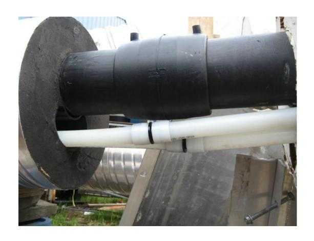
Photo 2: New glycol heat trace piping installed
