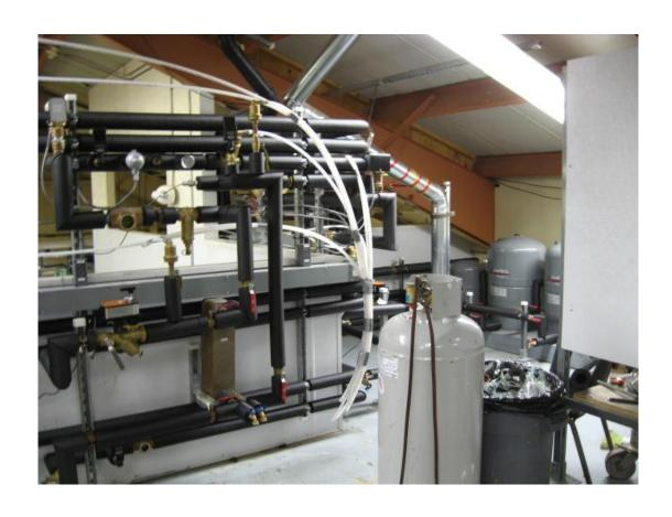
Photo 5: Hydronic heat add piping in the water treatment plant after insulation was installed
