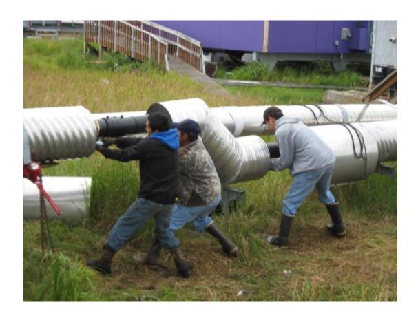
Photo 1: Selawik crew pulling new glycol lines on the vacuum sewer main
