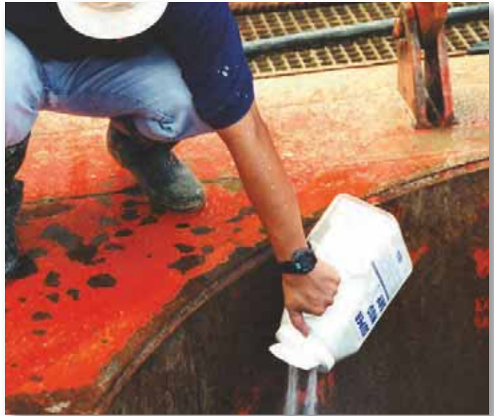
Mixing Directly into the Excavation
