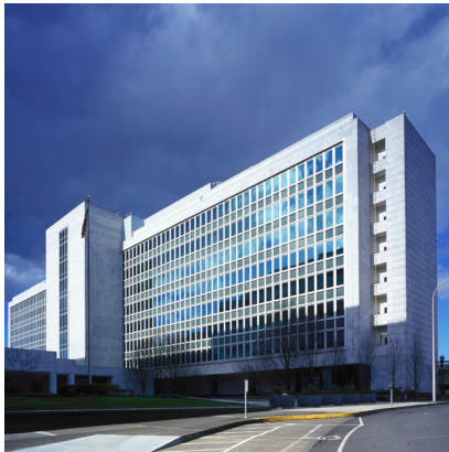
GSA 911 Federal Building
