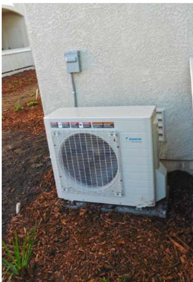
The air-to-water heat pumps provide efficient, combustion-free heating, cooling, and hot water.
