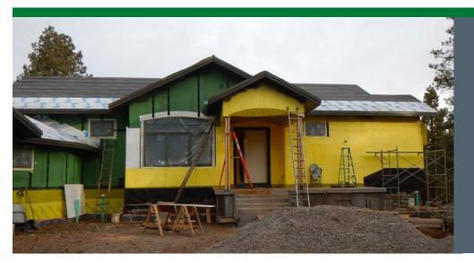
The 2x6 advanced framed walls were covered with a taped, coated sheathing and a mesh rain screen that provides a drainage plane and ventilation gap behind the stucco and stone exterior. Ice-and-water shield protects the edges and valleys of the roof while a three-layer vapor-permeable roof underlayment provides an air and water barrier. Standing seam metal roofing and 6.3 kW of solar panels were installed. The solar electric system should cut annual utility bills by \$2,600.
