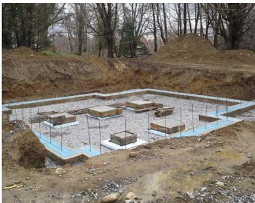
Four inches of rigid foam will wrap the slab perimeter while an additional 8 inches (R-35.6) of high-density EPS rigid foam will extend under the entire slab.
