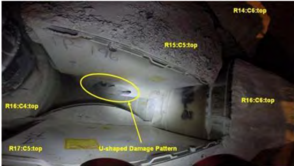
Figure 6-37: Damage to Slip Sheet at R15:C5
