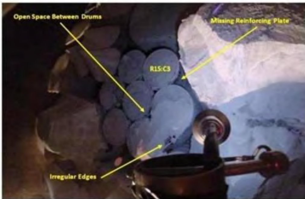
Figure 6-33: Missing Reinforcement Plate at R15:C3
