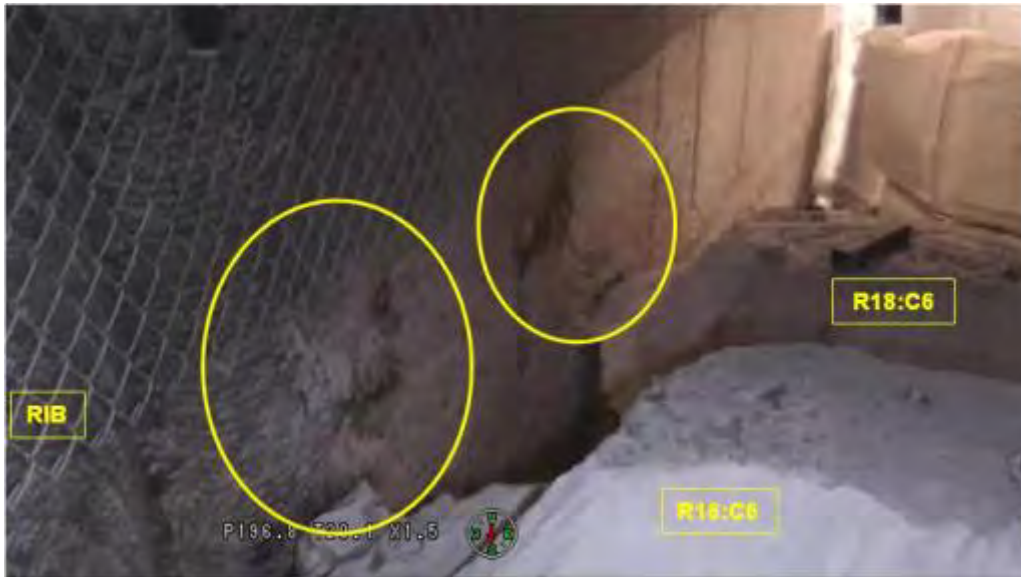
Figure 6-17: Rib Damage near Rows 16 and 18
