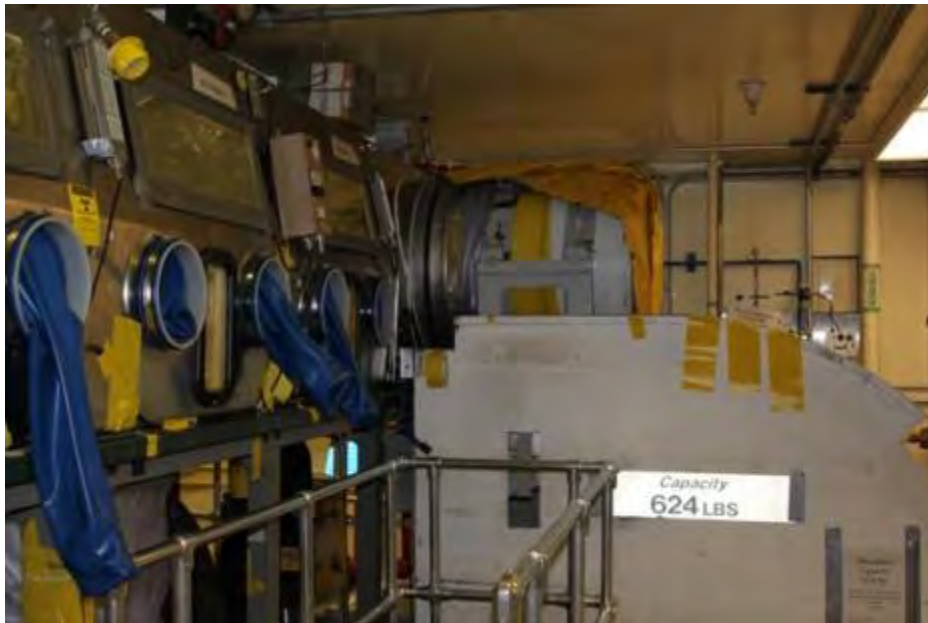
Figure 1-7: Waste Characterization Glovebox in WCRRF at LANL
