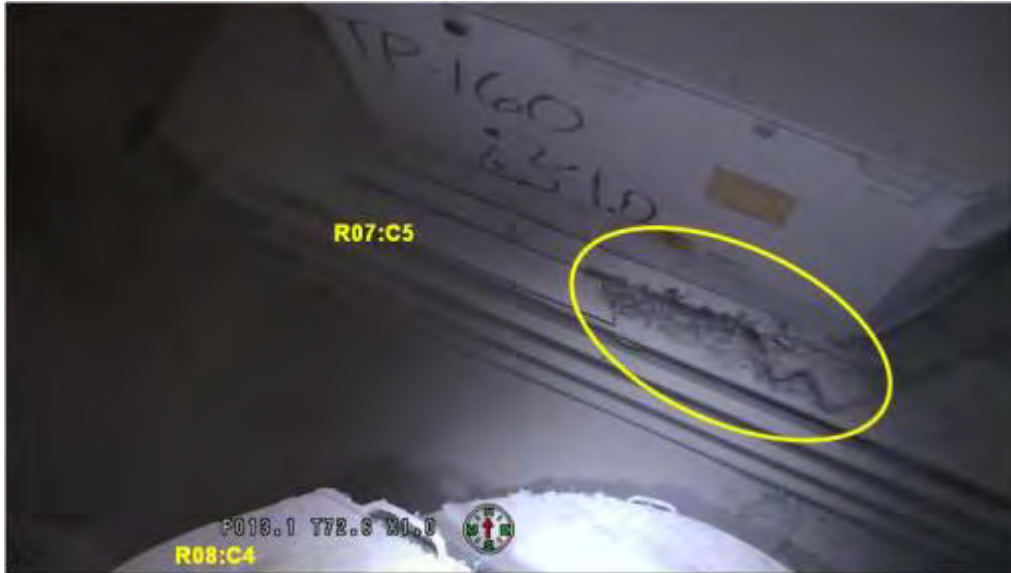
Figure 6-10: Fiberboard Slip Sheet Damage at R7:C5
