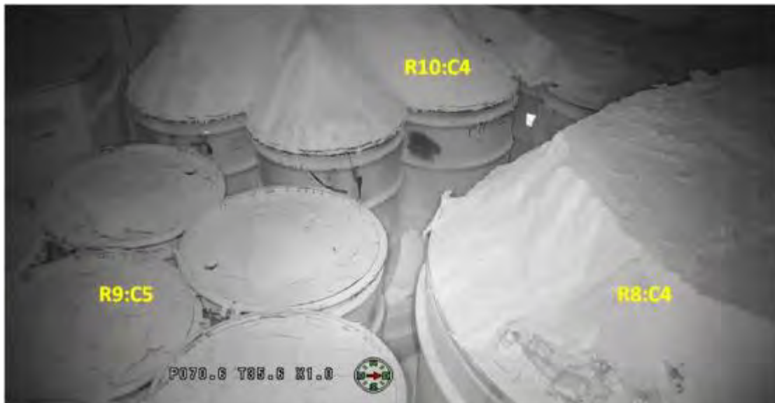
Figure 6-22: Damage at R9:C5 and R10:C4
