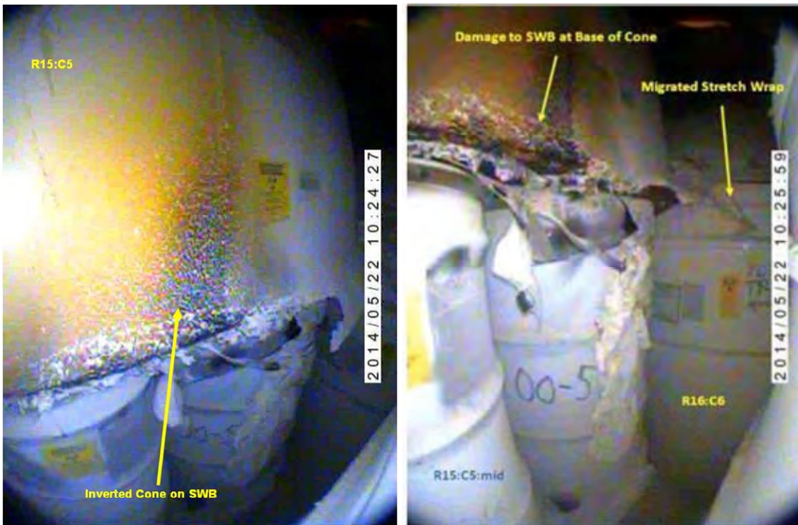
Figure 6-36: Side of SWB at R15:C5:top
