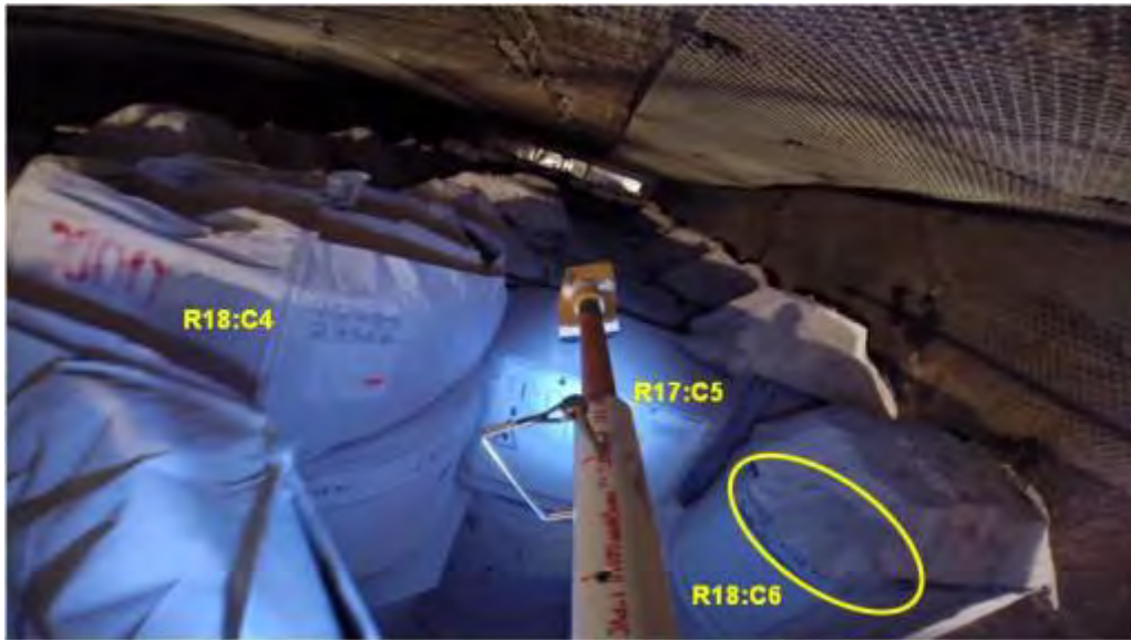
Figure 6-15: Cantilevered Bridge at R18:C6
