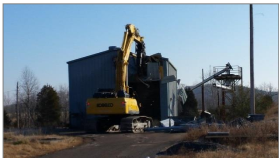
Demolition of K-892Y
