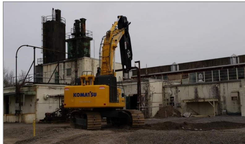
Demolition of K-892
