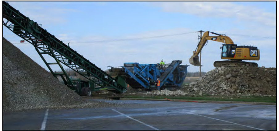
Rock crushing operation.
