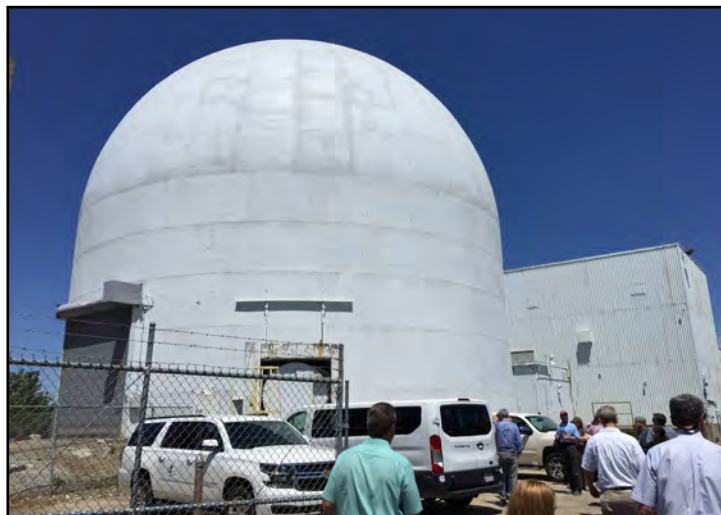
LM staff heading into the Piqua Decommissioned Nuclear Reactor.
