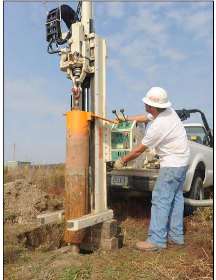
Self-performed well installations and abandonments are conducted using a Geoprobe® drilling machine.
