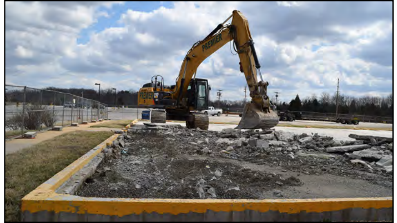
Foundation removal at the previously demolished administration building area.
