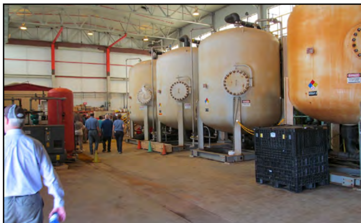
LM staff tour the Converted Advance Wastewater Treatment Facility at the Fernald Preserve.
