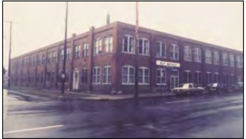
B&T Metals, in Columbus, extruded uranium rods for the Manhattan Project.
