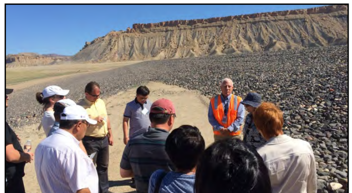
DOE Environmental Management staff describe the ongoing construction and waste disposal at the Moab project disposal site in Crescent Junction, Utah.
