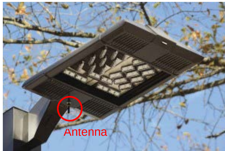
Figure 2-2: Example of a Controller integrated internal to a luminaire; note the small protruding antenna.
