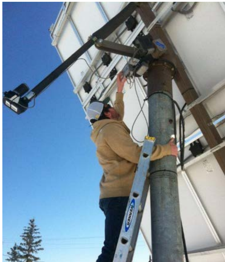
Photo by Brian Hirsch, NREL 20893
