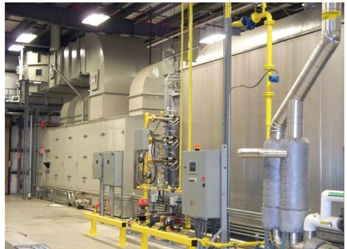
The CHP system is comprised of a Solar Centaur® 50 natural gas combustion turbine and a Rentech HRSG equipped with supplemental duct firing. *Photo credit Frito-Lay North America, Inc.*
