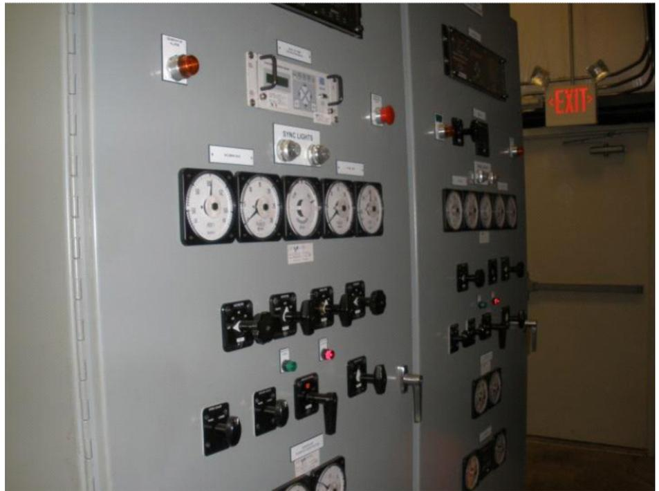
The Frito-Lay plant has electrical interconnect, including switchgear, primary power wiring, relays, etc., allowing power generation in parallel with Connecticut Light and Power's electrical grid. *Photo credit Frito-Lay North America, Inc.*
