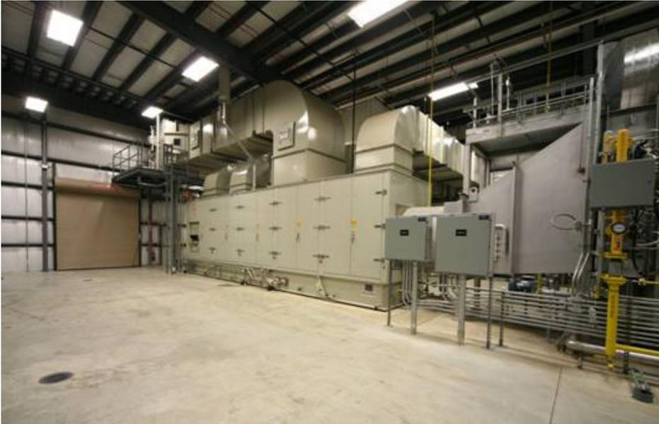
The CHP system was designed to be electric-load following and have the capacity to meet nearly 100% of the plant’s electrical power needs as well as the majority of the facility’s annual steam needs. *Photo credit Frito-Lay North America, Inc.*
