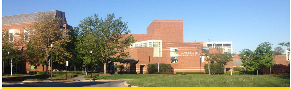
Exterior view of the University of Maryland Clarice Smith Performing Arts Center. The varying shapes and sizes hint at the diversity of the interior spaces.
