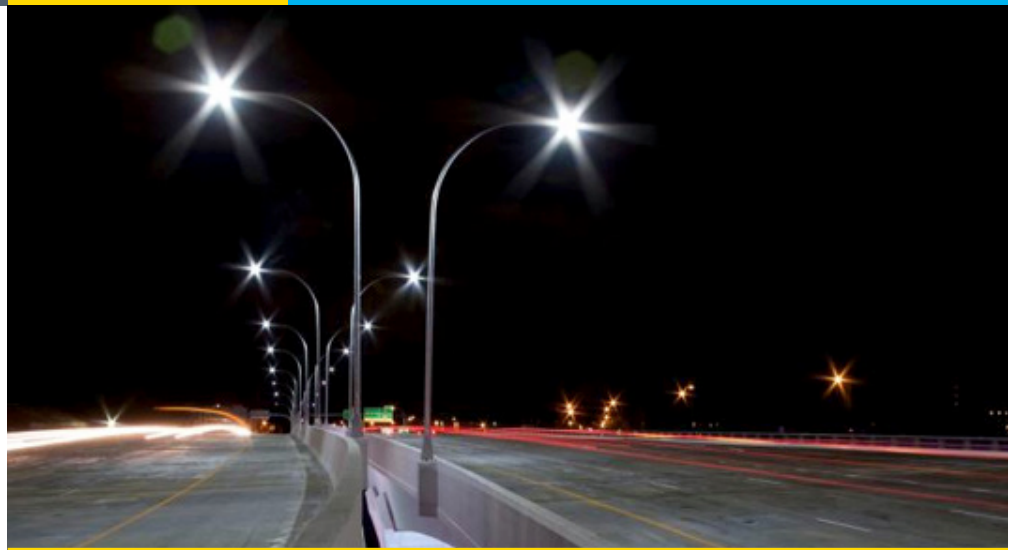
LED luminaires on the I-35W Bridge
